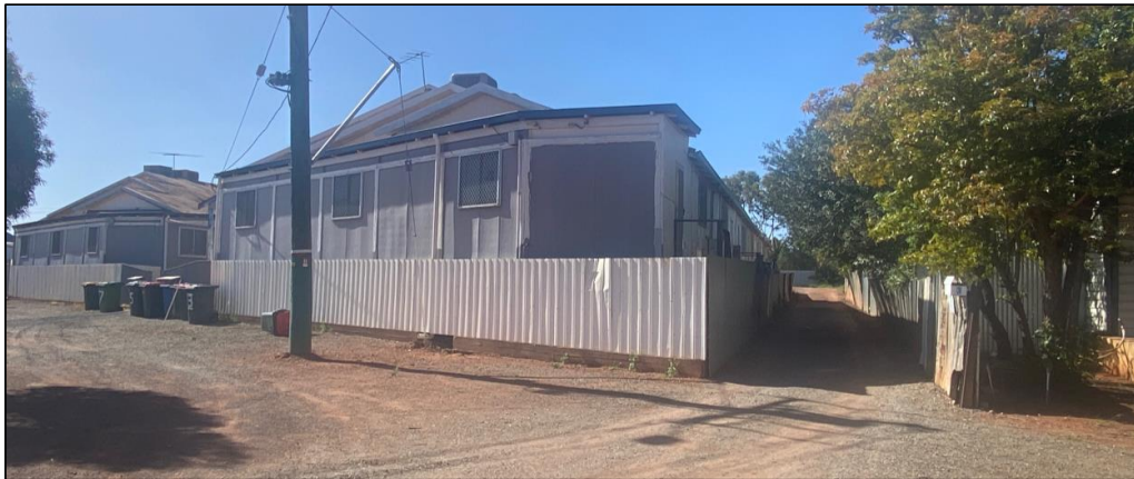
Photograph 2: Subject site and eastern ROW, as viewed from Porter Street looking north
