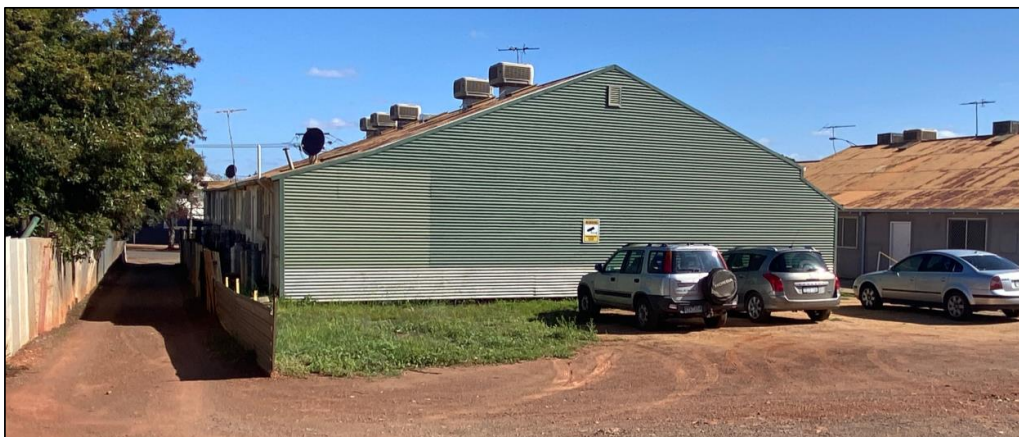
Photograph 4: Existing development, as viewed from rear of subject site looking south-west
