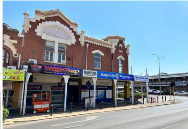
Figure 3 – Image taken September 2023, after completion
