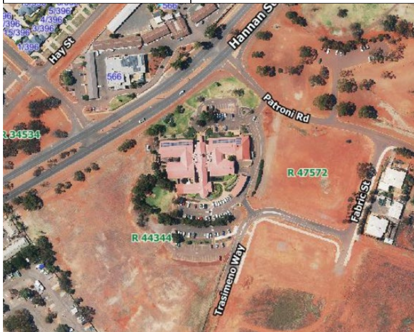
CKB Administrative Center 577 Hannan Street Somerville
