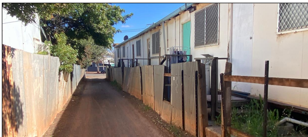
Photograph 3: Eastern ROW and subject site, looking south
