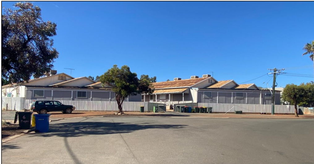
Photograph 1: Subject site, as viewed from Porter Street looking north-east
