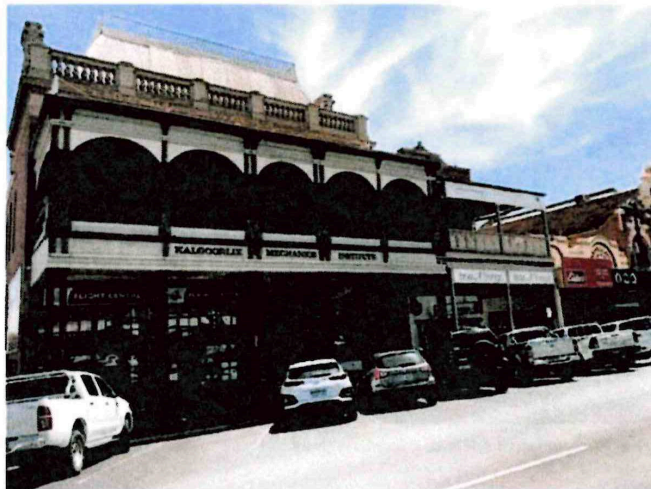
Figure 2: Photograph of the Mechanics Institute (fmr)
